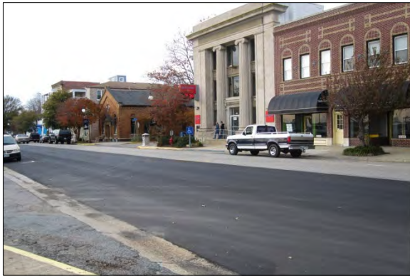
Photo 3 - 182-0002 - Cape Charles Historic District Mason Avenue
