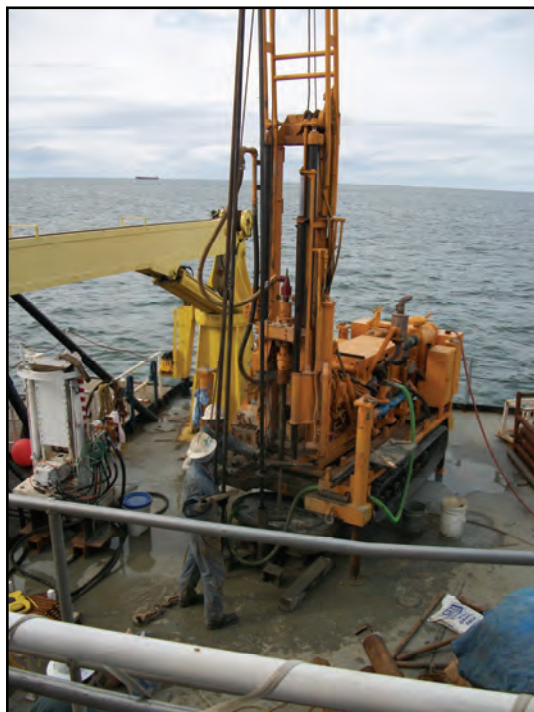
Track Mounted Drill Rig (orange) for Deep Borings
