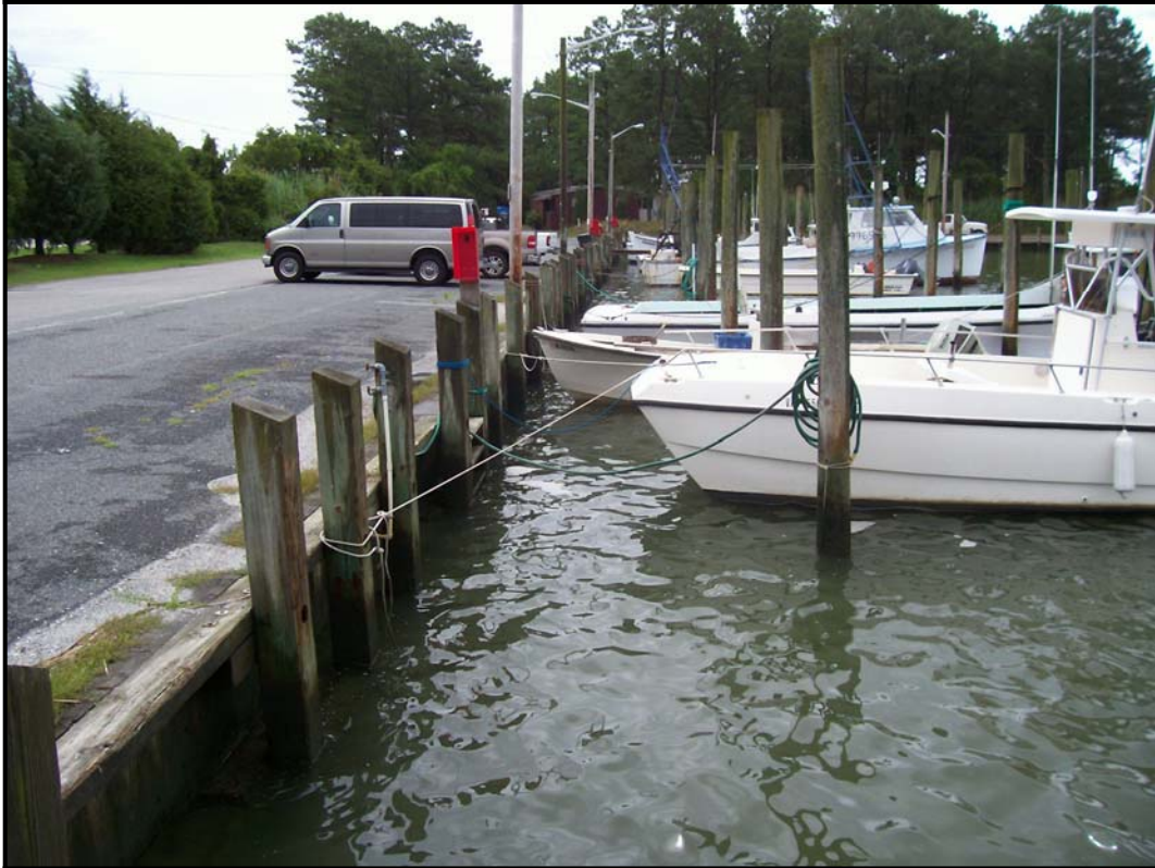
Site Photograph 3. Typical condition of the harbor's 20-year-old bulkhead.
