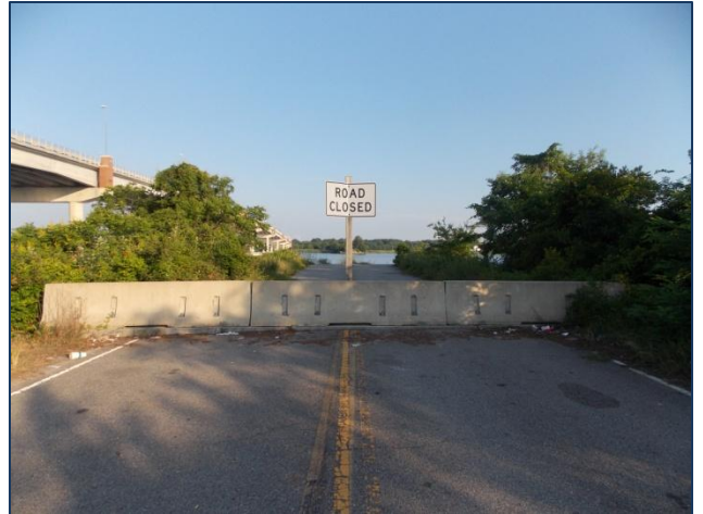
Second road barrier at the sight.
