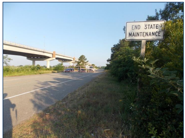
Photo from property line. The road terminus at F-600.
