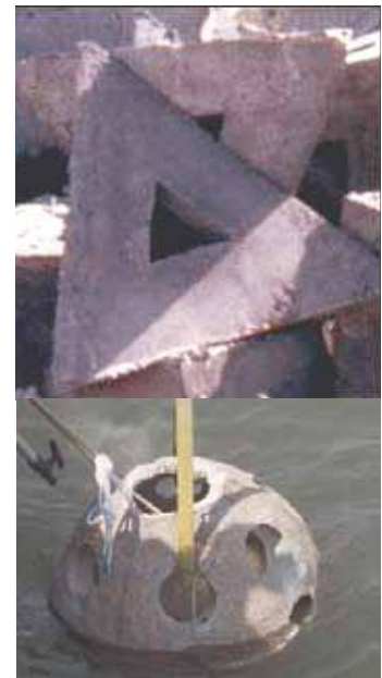
Tetrahedrons (top) and deployment of a reef ball (bottom).
