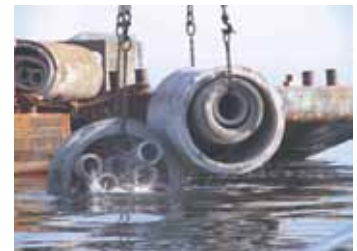
Pipe being lowered to form an artificial fishing reef.
