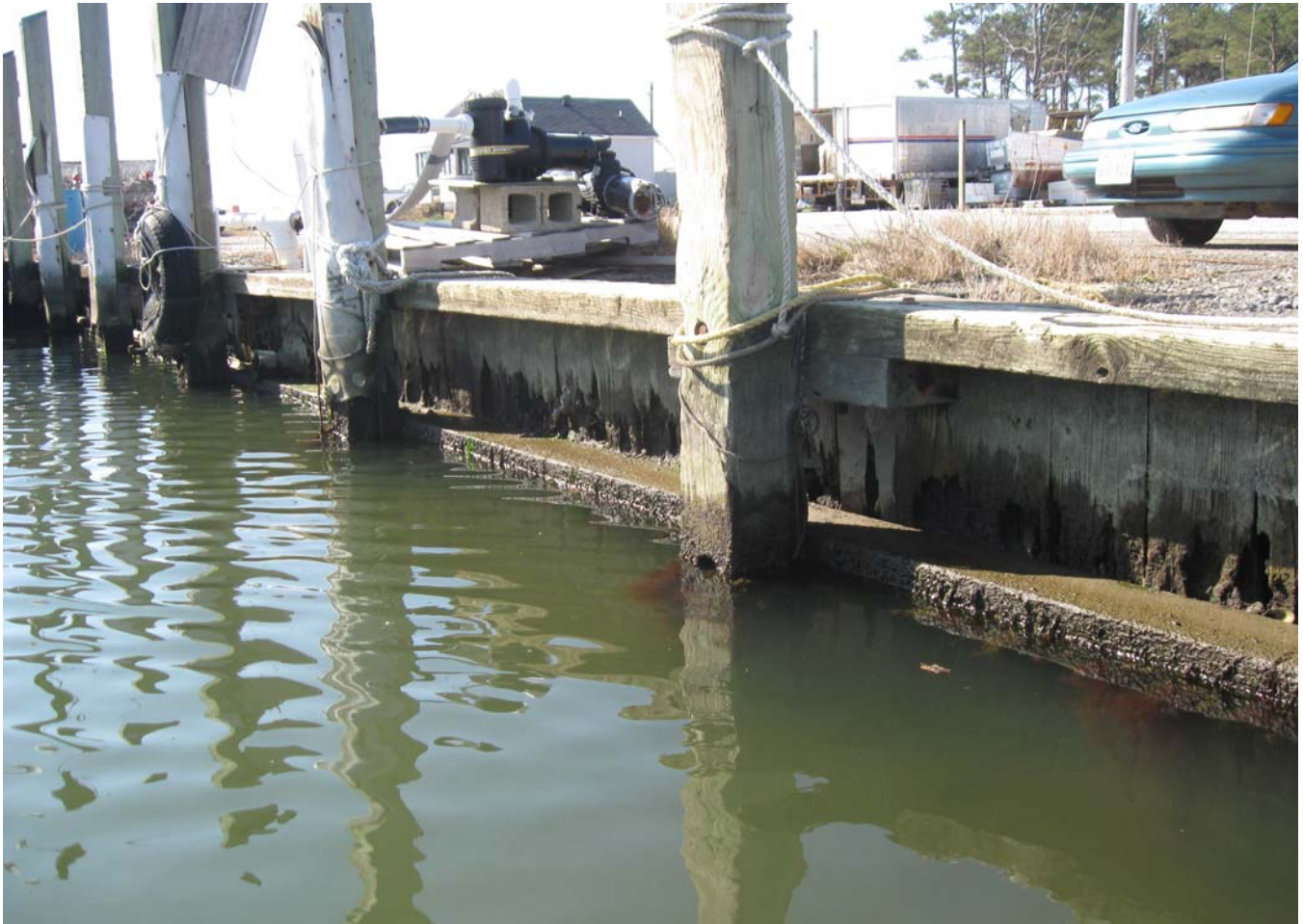
DETERIORATED TIMBER SHEETING
