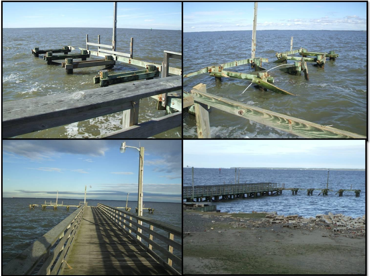
Figure 1. The Saxis Municipal Pier one day after Hurricane Sandy (10/31/12).
