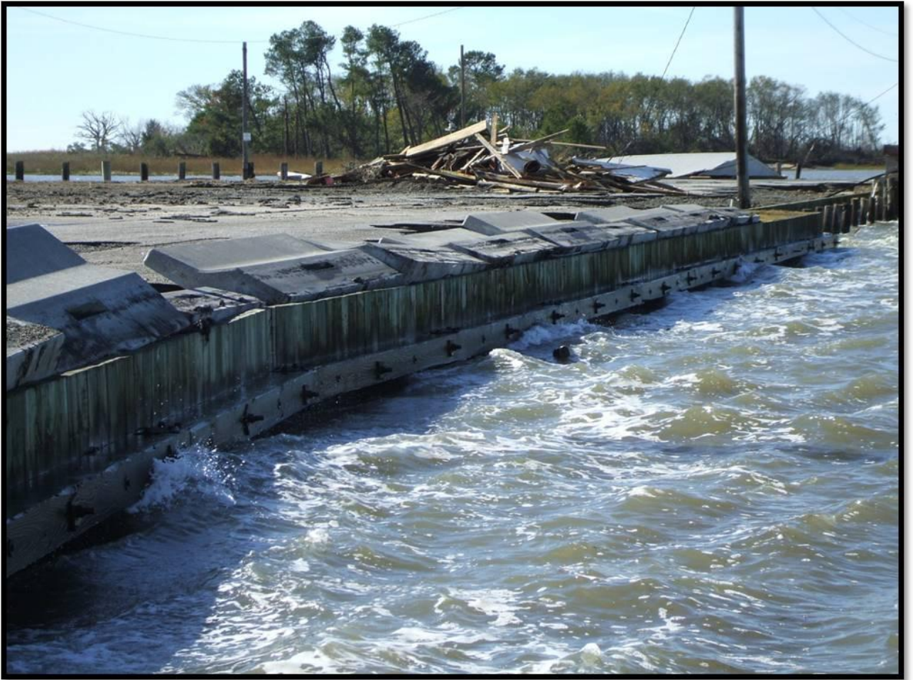
Figure 2. Evidence of the wave forces experienced at the Saxis Municipal Pier during and after Hurricane Sandy (10/31/12).
